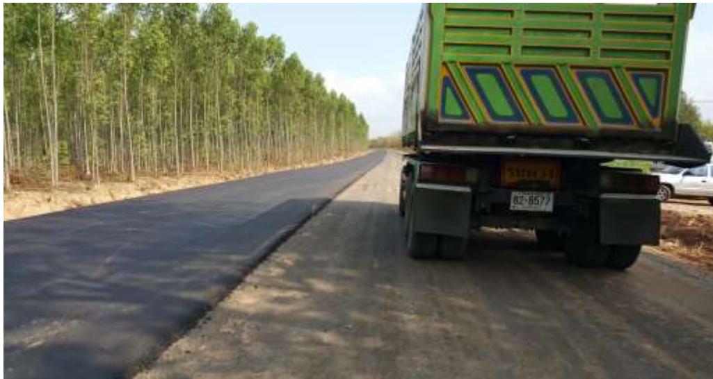
Rubberised road project at Chachoengsao, Thailand
